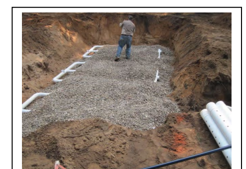
Figure 9: Backfilling of drainfield
