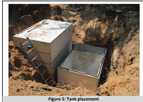
Figure 5: Tank placement
