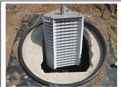
Figure 7: Oversized effluent filter. Tank access cover needed to be widened to allow for installation of filter
