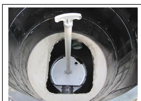
Figure 8: Oversized effluent filter and tank access riser brought to grade.
