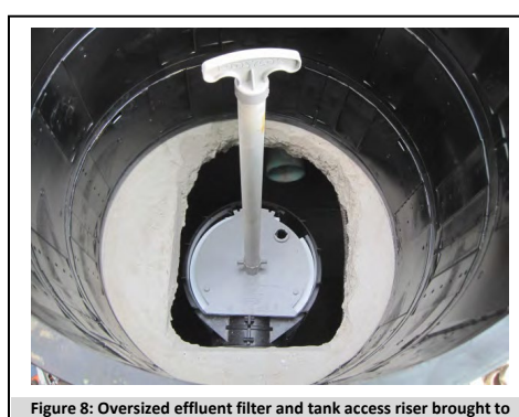
Figure 8: Oversized effluent filter and tank access riser brought to grade
