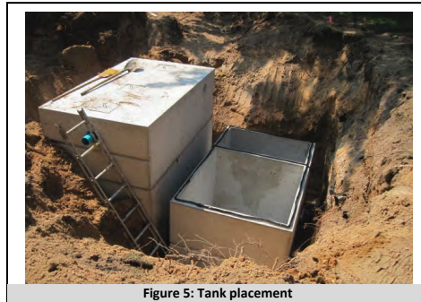
Figure 5: Tank placement
