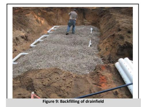
Figure 9: Backfilling of drainfield
