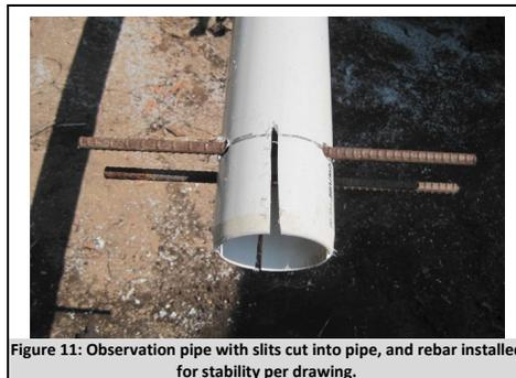
Figure 11: Observation pipe with slits cut into pipe, and rebar installed for stability per drawing.
