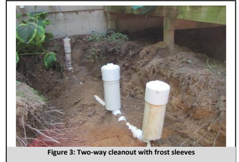
Figure 3: Two-way cleanout with frost sleeves
