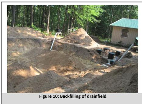
Figure 10: Backfilling of drainfield
