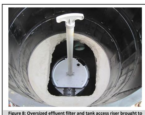
Figure 8: Oversized effluent filter and tank access riser brought to grade.
