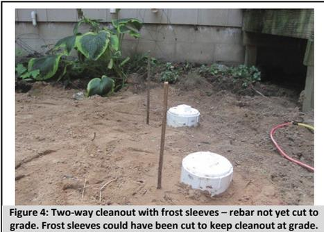
Figure 4: Two-way cleanout with frost sleeves – rebar not yet cut to grade. Frost sleeves could have been cut to keep cleanout at grade.
