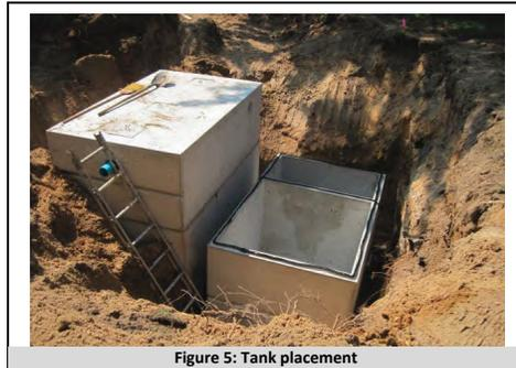
Figure 5: Tank placement
