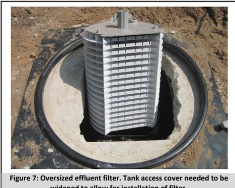
Figure 7: Oversized effluent filter. Tank access cover needed to be widened to allow for installation of filter
