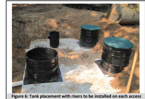
Figure 6: Tank placement with risers to be installed on each access port and brought to grade.
