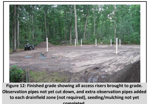
Figure 12: Finished grade showing all access risers brought to grade. Observation pipes not yet cut down, and extra observation pipes added to each drainfield zone (not required), seeding/mulching not yet completed.
