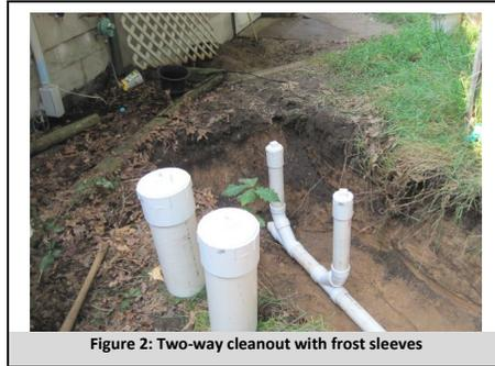
Figure 2: Two-way cleanout with frost sleeves
